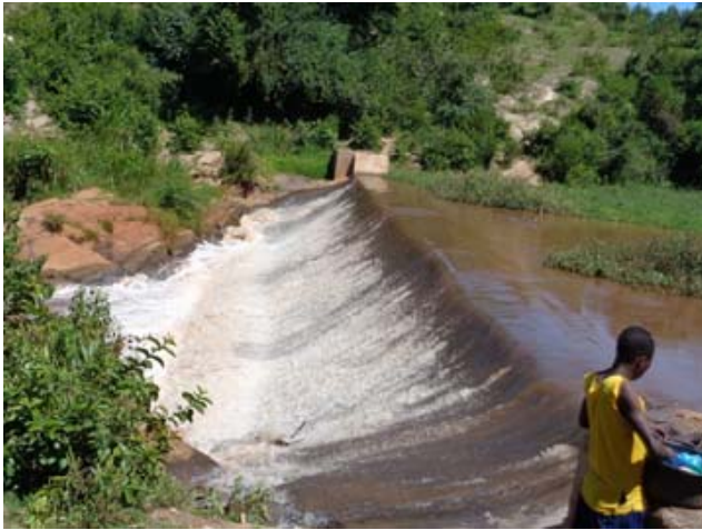
Photo Plate 5: Silt trap constructed across Kibisi River
