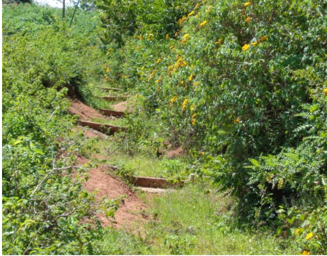
Photo Plate 2: Erosion protection along the roads
