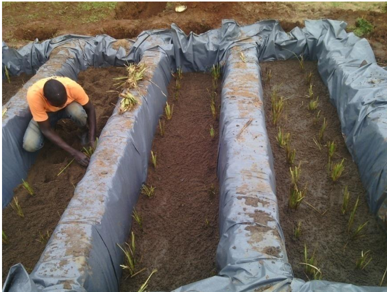
Plate 1: Planting of Vetiver grass slips
