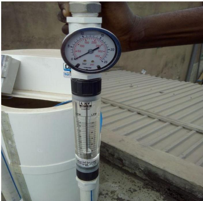
Pressure gauge installed on the water pumping system
