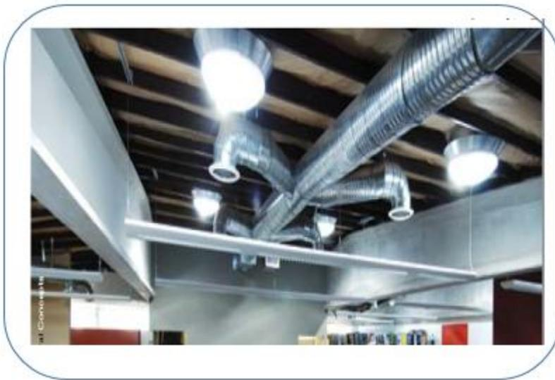
**Figure 4.5: Light pipe Distribution Network**
