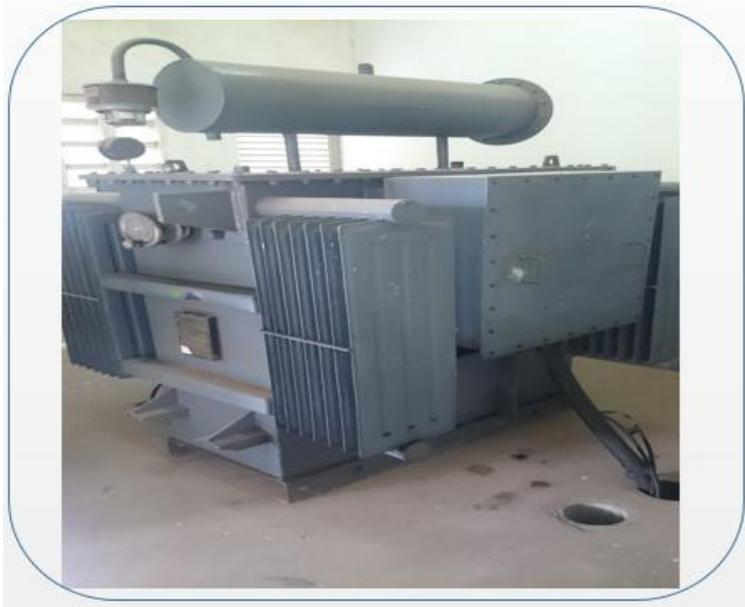
**Figure 1.2: 630KVA Transformer serving Equatorial Fidelity Centre**
