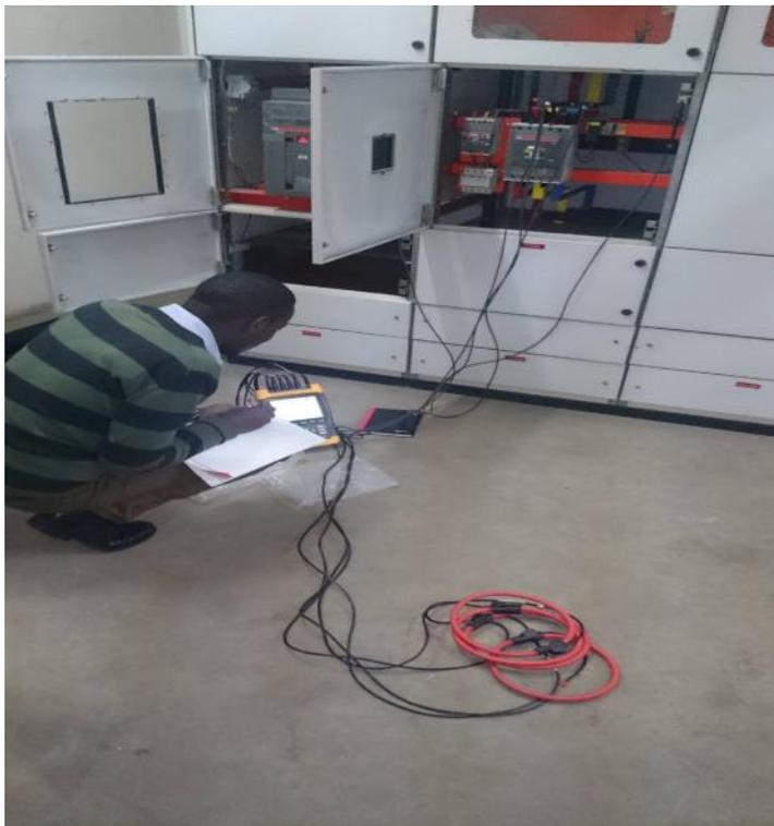
Fig 4.3: Power analysis from the bus bars
