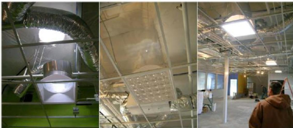
**Fig 2.14: Light pipe serving four under-ground floors**
