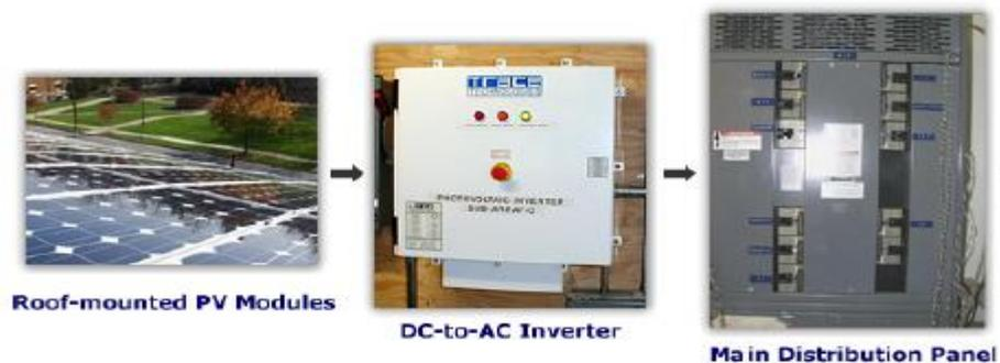
**Fig 2.3: Major components in Installation of solar PV**
