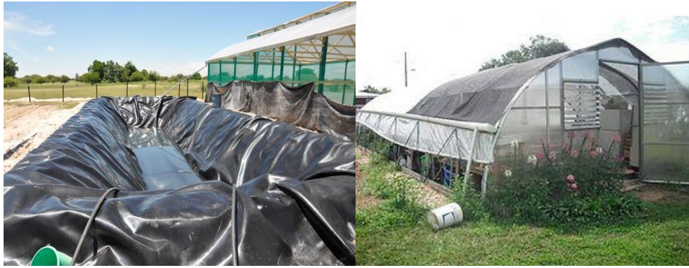
Figure 3: Greenhouse Rooftop and collection ditch
