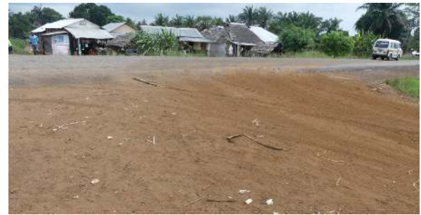
Side road (unpaved) intersection at Bwiti Junction (gate 02, Fig. 5.4) illustrating exposed road murrum.
