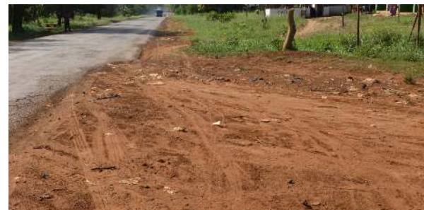
Mrima TM Junction roadside bus stop (gate 01, Fig. 5.5 b) illustrating exposed road murrum.
