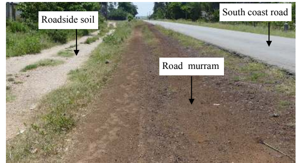
South coast paved road toward Ramisi. Illustrating difference between road murrum and roadside soil.
