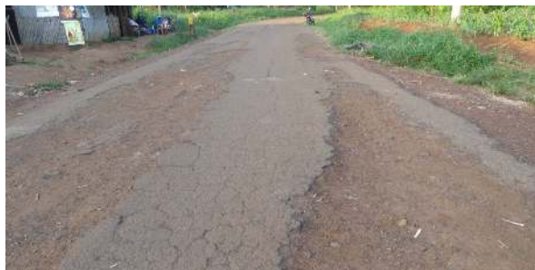
Side paved road intersection at Mrima TM Junction (gate 03, Fig. 5.5 b) illustrating weathered tarmac.
