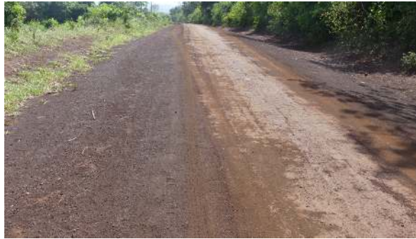
Dry weather murram road at the base of Mrima Hill. Also illustrated is the weathering and run-off of top soil.
