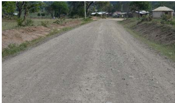
Dry weather murram road in Menzamwenye, east of Mrima Hill. Also illustrated is the difference in soil type.
