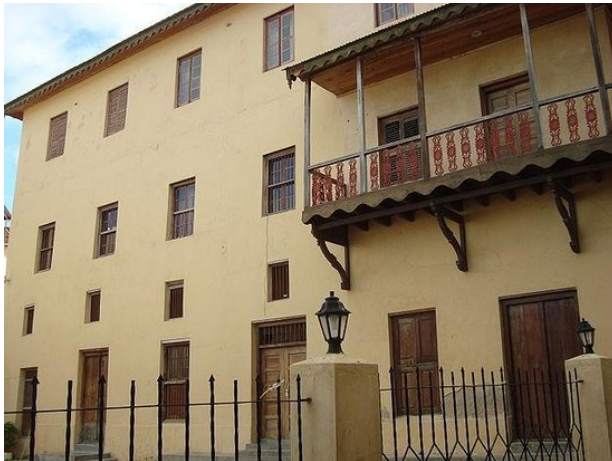
Fig 2- 15: Leven House is an example of a retained facade as it is protected under the conservation act in Kenya. The new facade mimics exactly the original building. Although the original building was almost a ruin, it was restored. Source: Author
