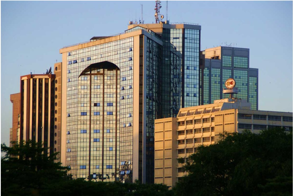
Fig 3-3: View Park towers view from Central Park at sunset. This skyscraper was amongst the first to be built in Kenya. It is surrounded by Hazina Towers on the left, Ambank house at the back and Utalii House on the right. Source: Author
