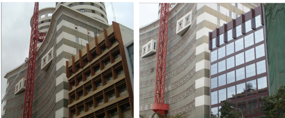
Fig 2- 13: Victor house as originally built on the left and glass cladded (2014) on the right. Source: Musau Kimeu, July 2015
