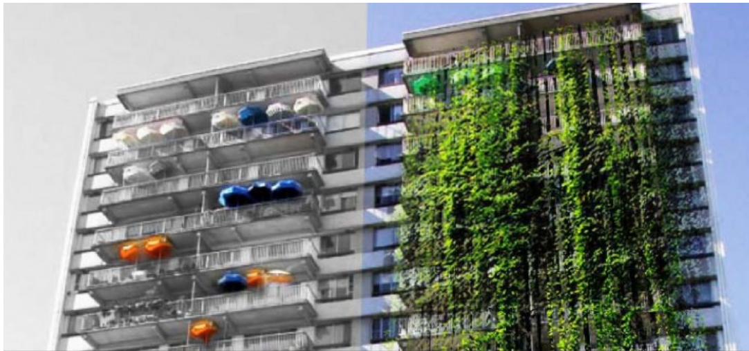
Fig 2-8: A building envelope which is existing can be improved by changing the building envelope so that the thermal; performance of the building can increase. Source: Arch Laura Pedata, Tirana, Polis University (2011)
