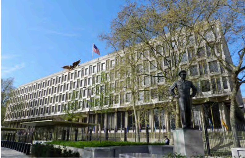
Plate 2.7: The American Embassy in London after Fortification
