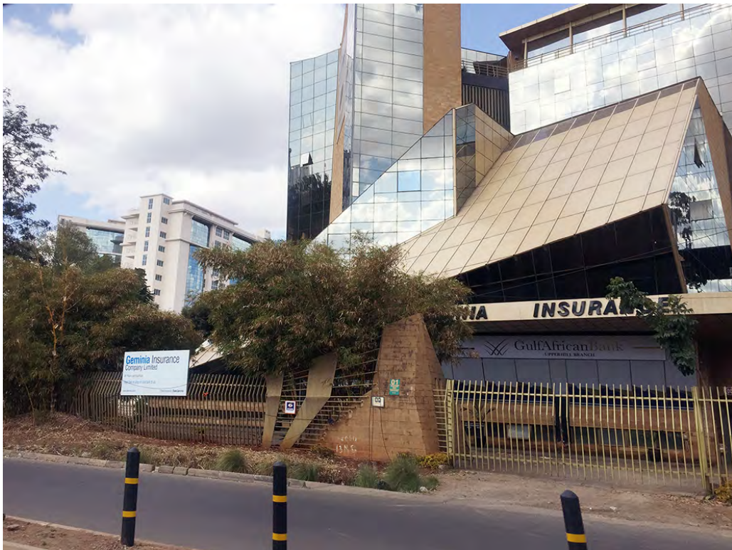
Plate 4.12: A Porous Wall to a building in Upper Hill
