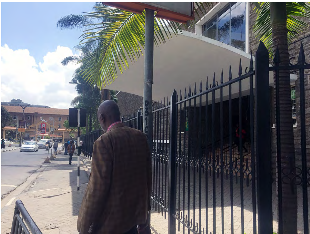
Plate 4.27: The County Offices cordoning off a Public Street
