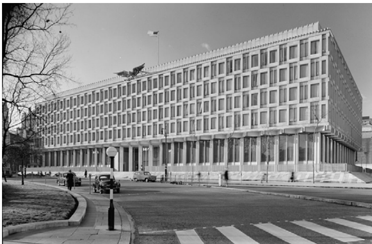
Plate 2.6: The American Embassy in London before Fortification
