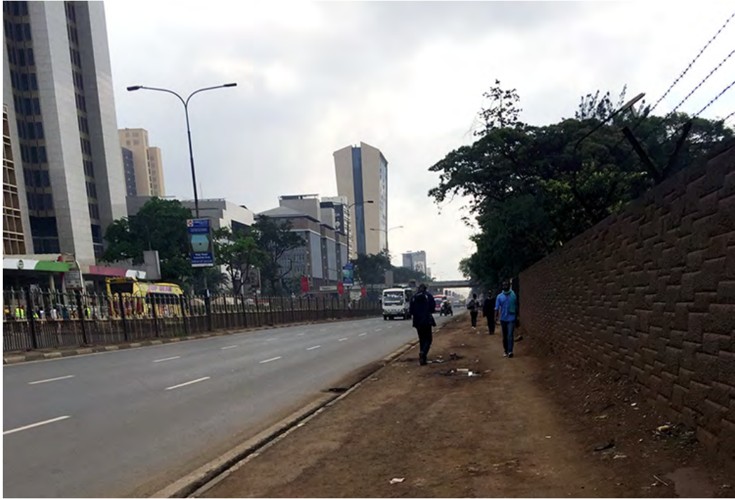
Plate 4.11: Boundary Wall to the Government Press along Haille Sellasie Avenue
