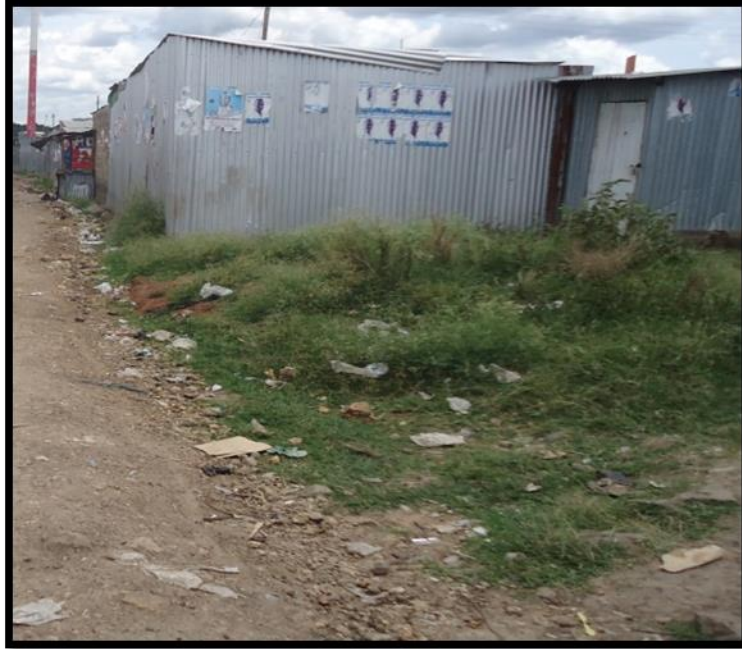
Figure 5. 5: Semi-Permanent House in KCC Village (Source: Author's field survey, 2017)
