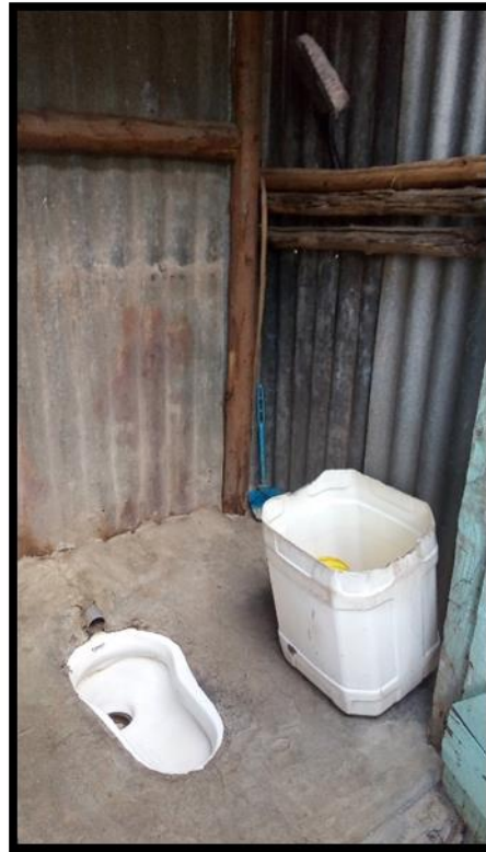
Figure 5.7: NCWSC Toilet Facility (Source: Author's field survey, 2017)
