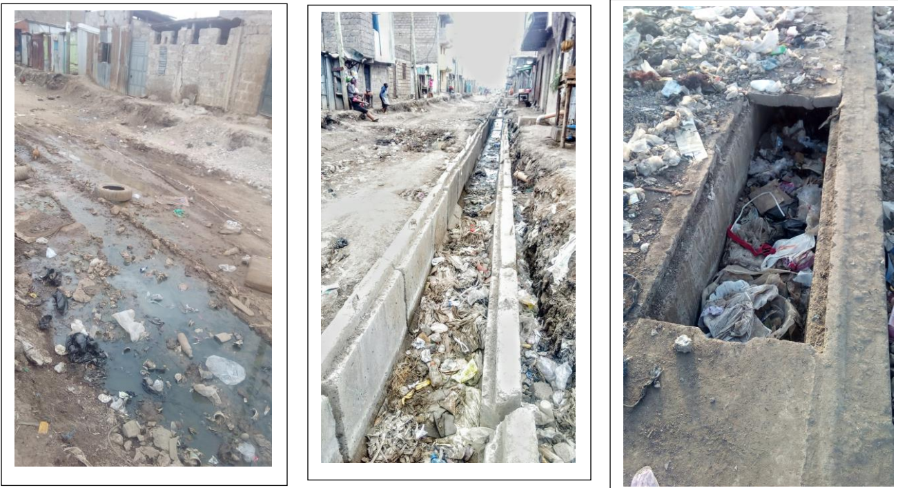
Figure 5.10 Condition of Drainage Structures
