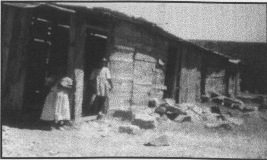
Plate No.3: Temporary structure
