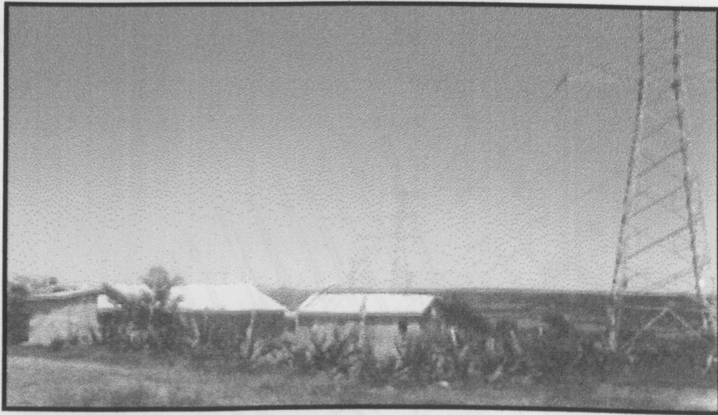
Plate No.8: An electrical pole located on the playground of P.C.G School
