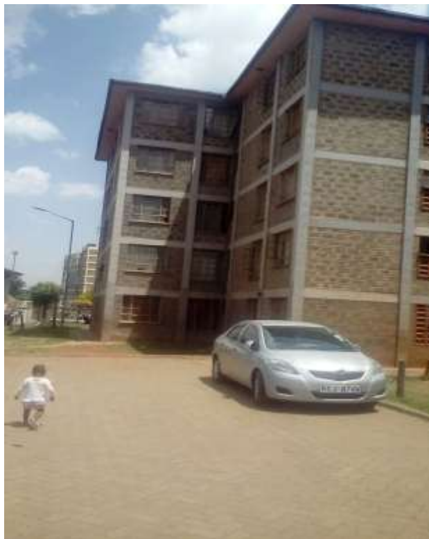
Side View of a Typical Flat at Jogoo Road Housing
