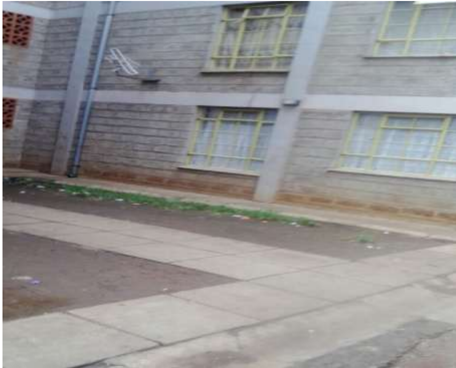
Rear View of a Typical Flat at Shauri Moyo Housing
