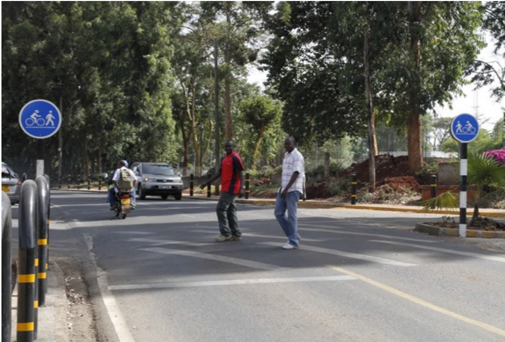
Plate 2-4: Raised pedestrian crosswalks at key crossing points
