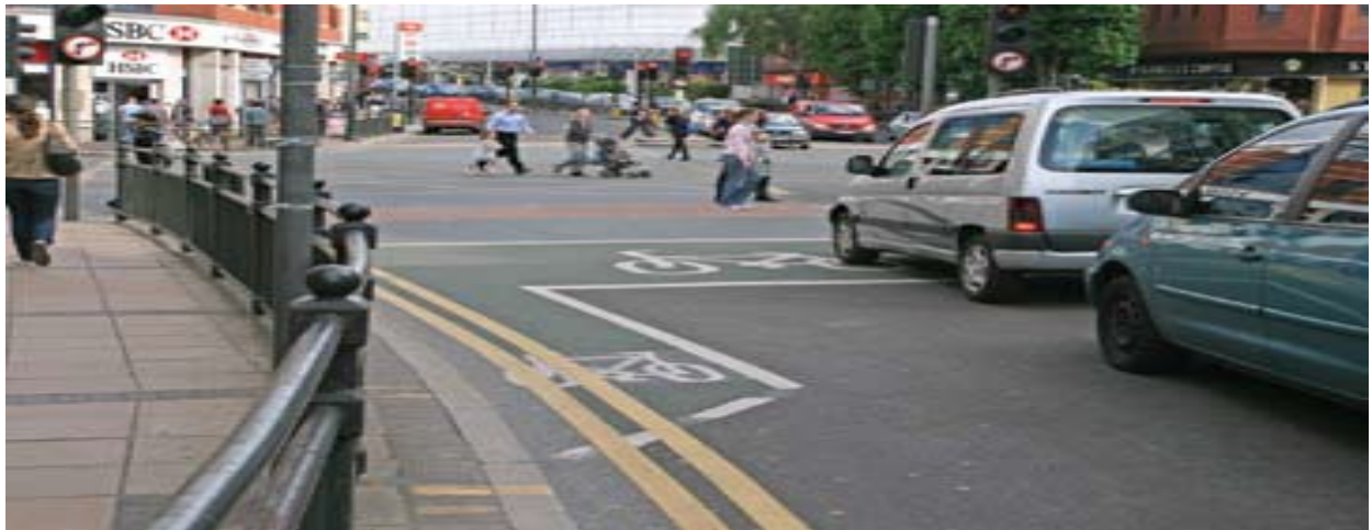
Figure 6–4: Railing used to direct pedestrians to crossing locations in London, UK
