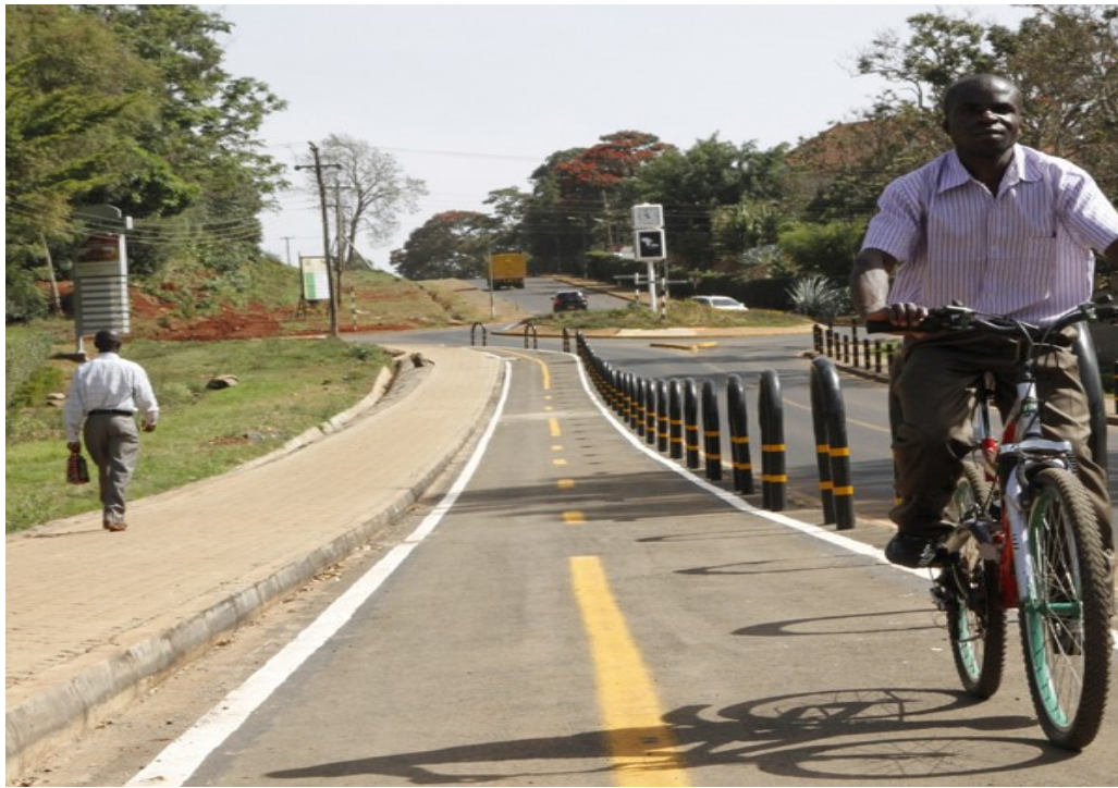
Plate 2-2: UN Avenue after rehabilitation
