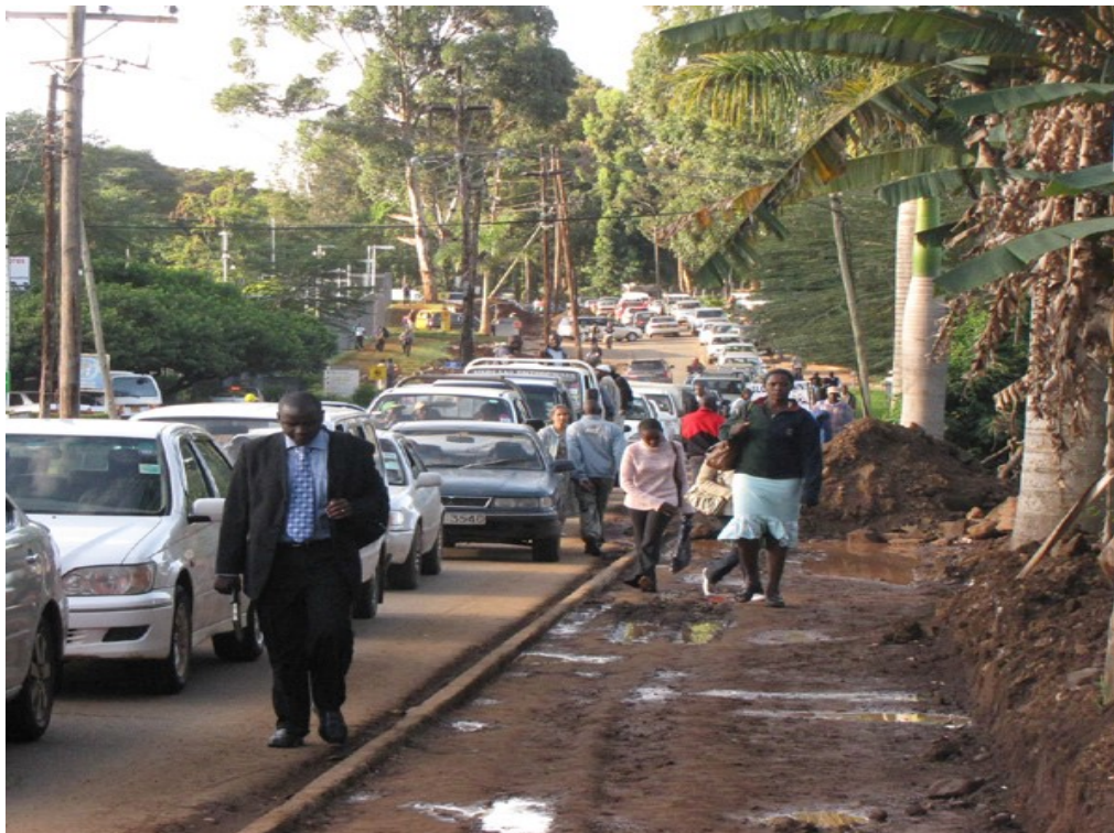
Plate 2-1: UN Avenue before rehabilitation
