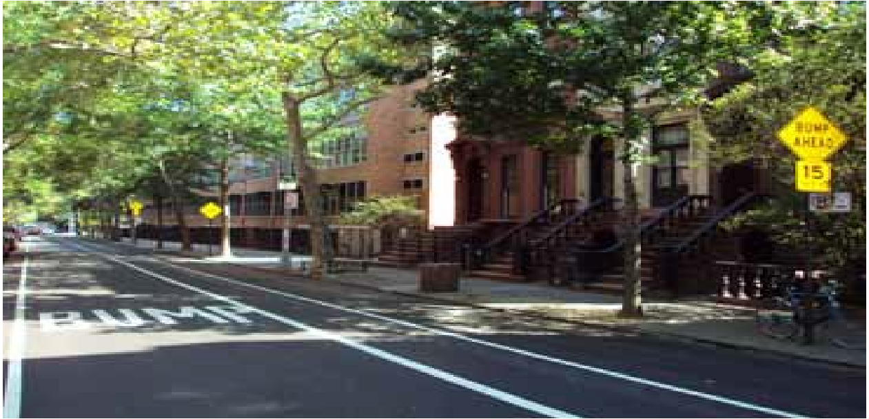
Figure 6–6: Speed reducers and road signs
