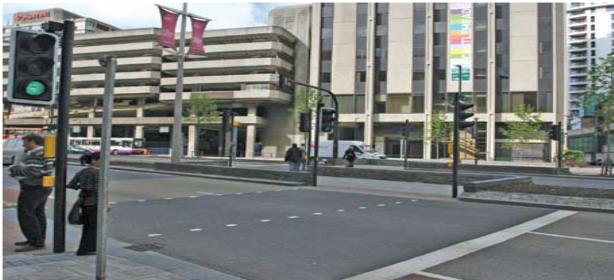
Figure 6–8: Offset pedestrian crossing at a signalized intersection in Bristol, UK.
