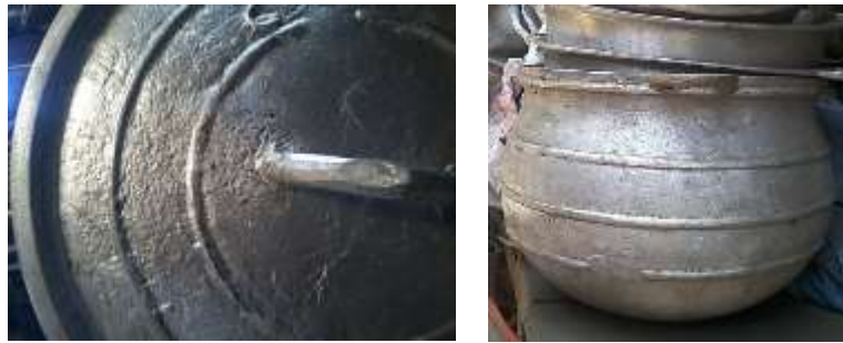
Figure 38: Inconsistent decorative ridges on the spherical boiling pot girth and lid
