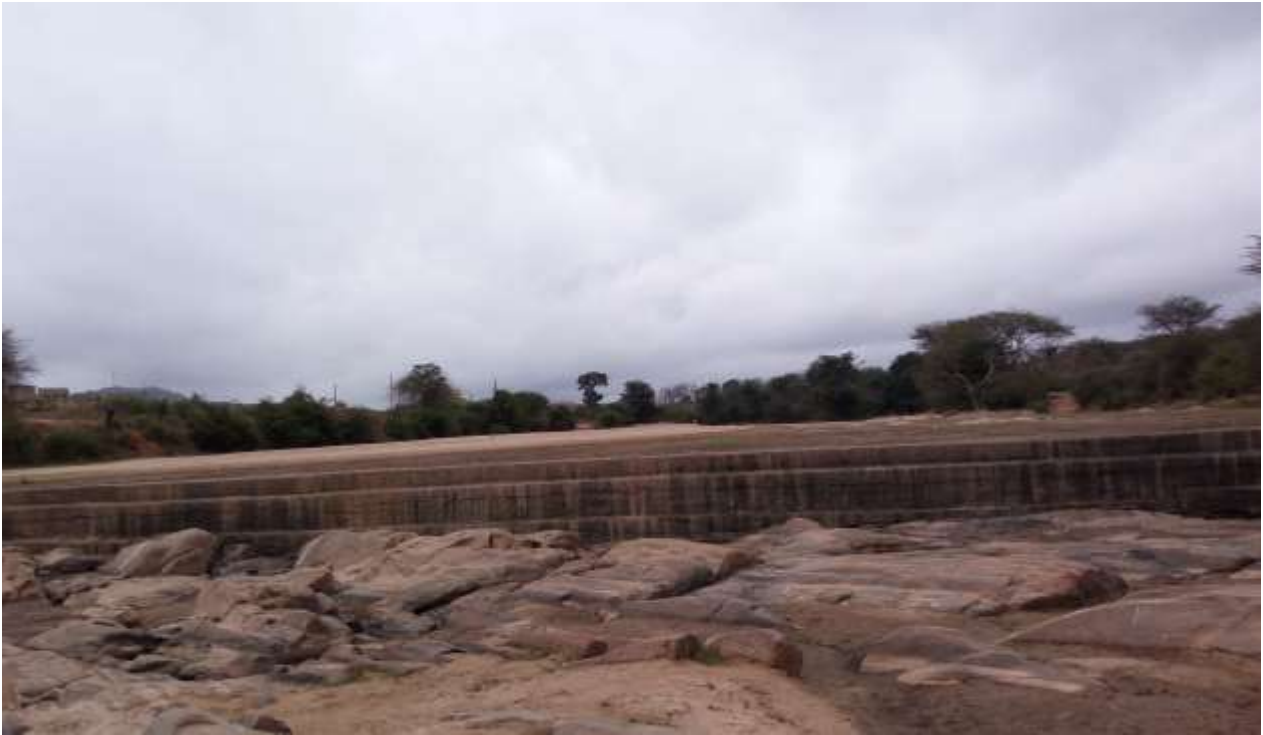
Plate 7-1: Kaiti Sand Dam
