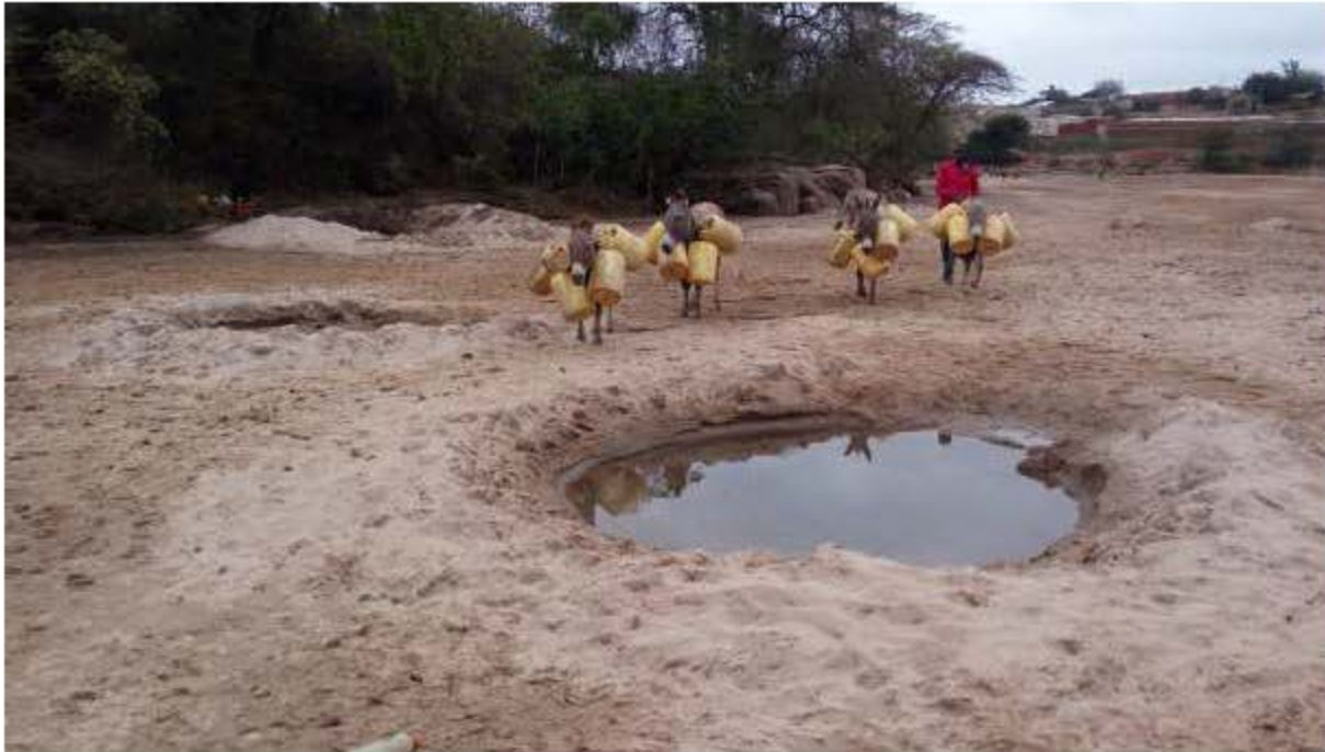
Plate 2-3: Scoop holes, Kaiti Sand Dam, Makueni County
