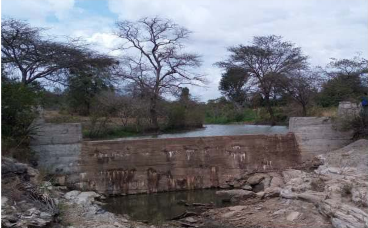
Plate 2-1: Immature Sand Dam, Vinya Wa Mwau Sand Dam, Makueni County
