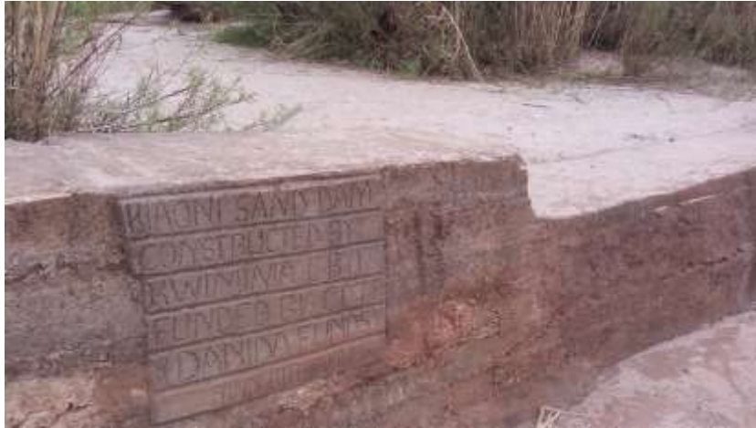
Plate 7-5: Kiaoni Sand Dam
