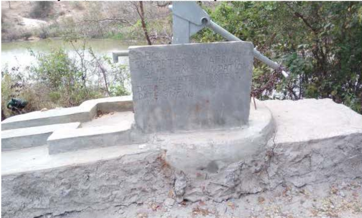
Plate 2-4: Shallow Well Hand Pump, Vinya Wa Mwau Sand Dam, Makueni County
