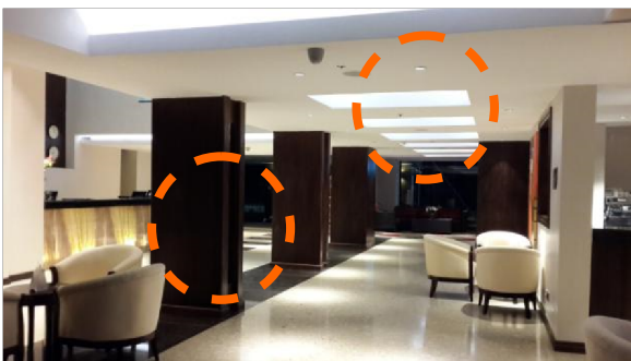
Fig 4.22 Lobby ceiling and columns
