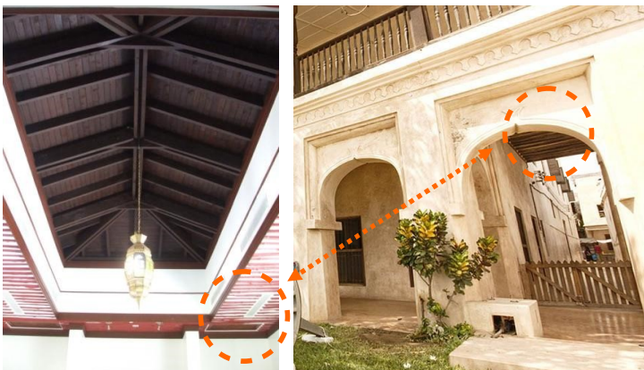
Fig 4.15a Ceiling with boriti poles (MSH) Fig 4.15b Ceiling with boriti poles (LM) Source: Planning Interiors Limited and Lamu Museum (NMK)
