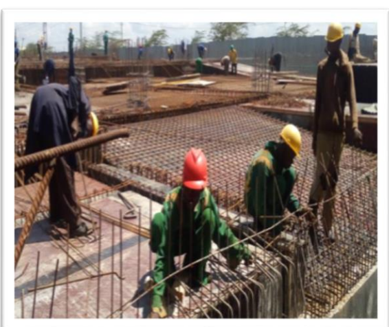
Steel worker tying reinforcement bars
