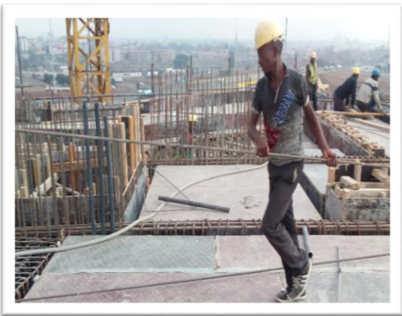
Steel worker carrying steel bar without PPE
