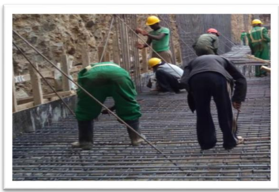
Steel worker carrying steel bar without PPE
