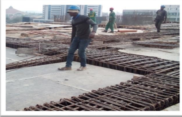
Steel worker tying reinforcement bars
