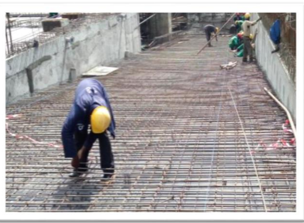
Steel worker tying reinforcement bars
