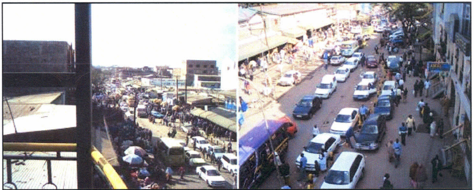
Plate 15: An aerial view of vehicle, pedestrian and hawking conflicts on First Avenue.
