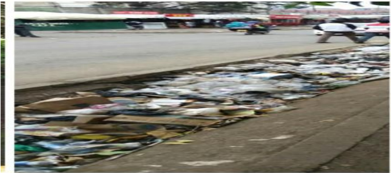
A trench in Kibra clogged with waste.
