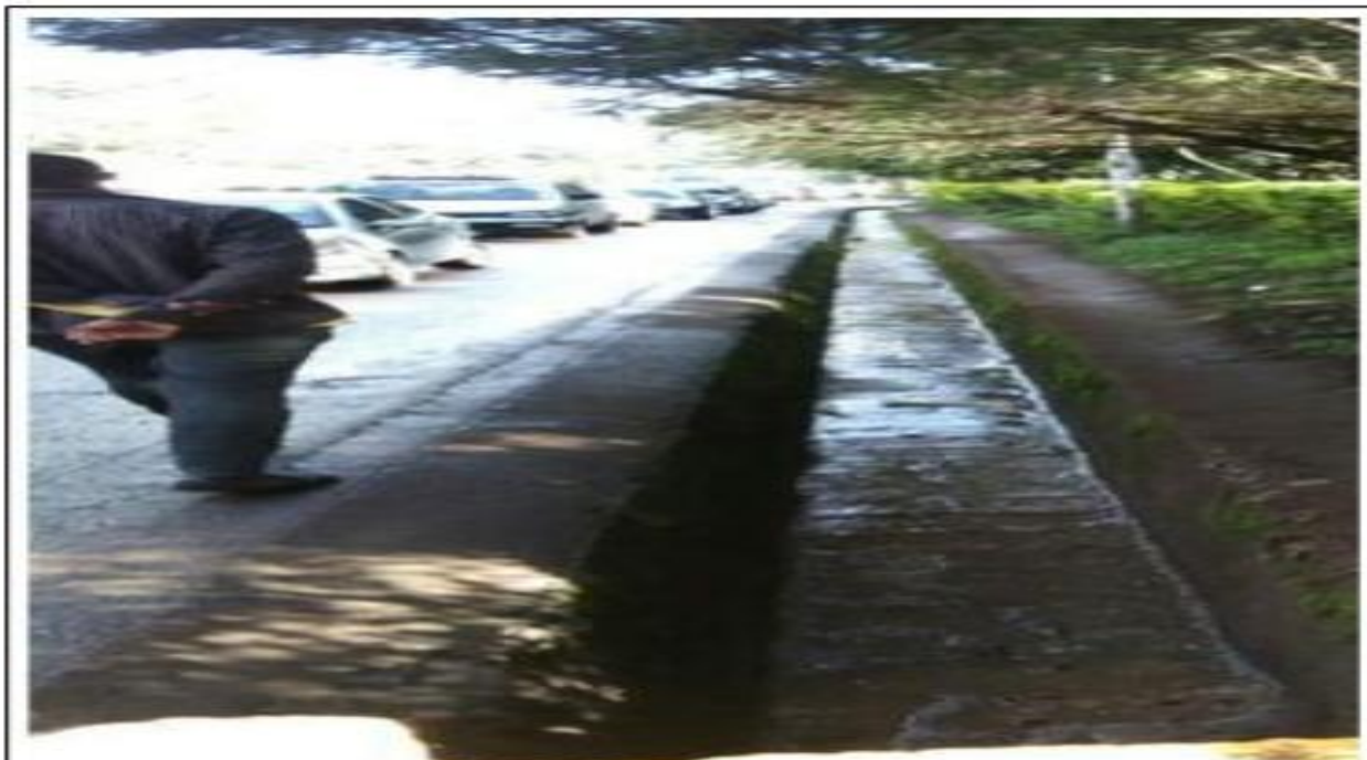
A trench at Lavington upper class zone, not clogged with waste.
