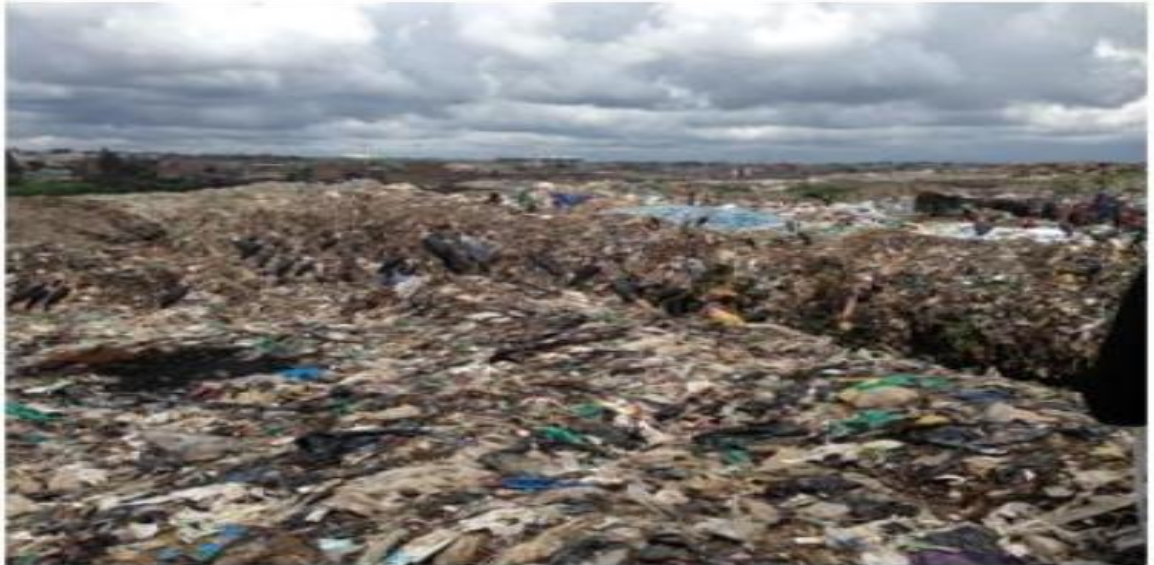
Open dumpsite at Dandora, contravenes the ten minimum requirements of National solid waste management Strategy of 2015, set by NEMA of a good landfill
