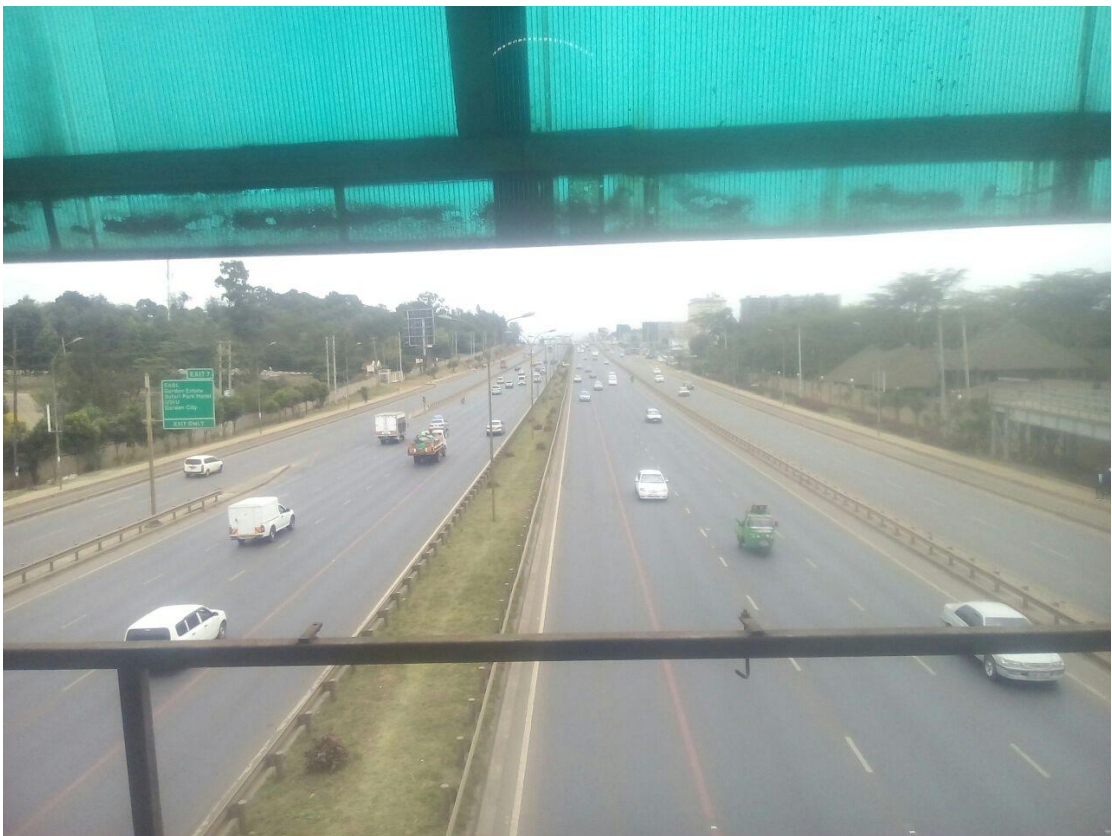
Plate 5.3 Eight Lane Highway Between Garden City and Roysambu Intersections Field Survey (2017)
