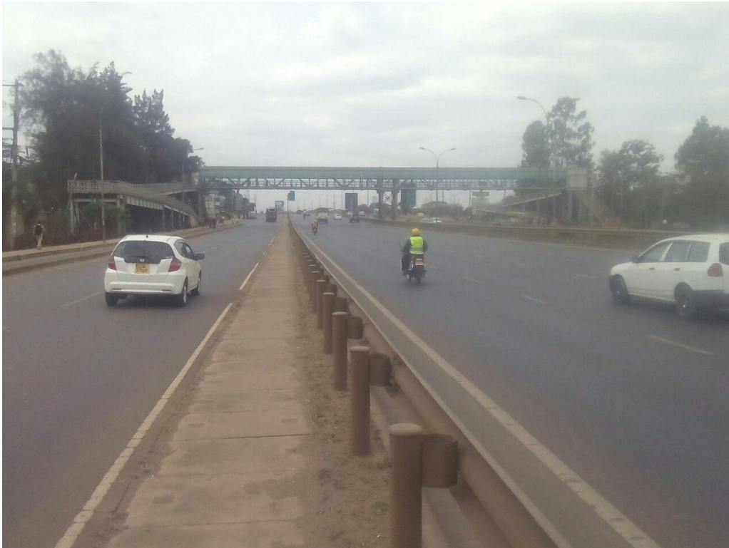
Plate 5.6 USIU Footbridge Field Survey (2017)
