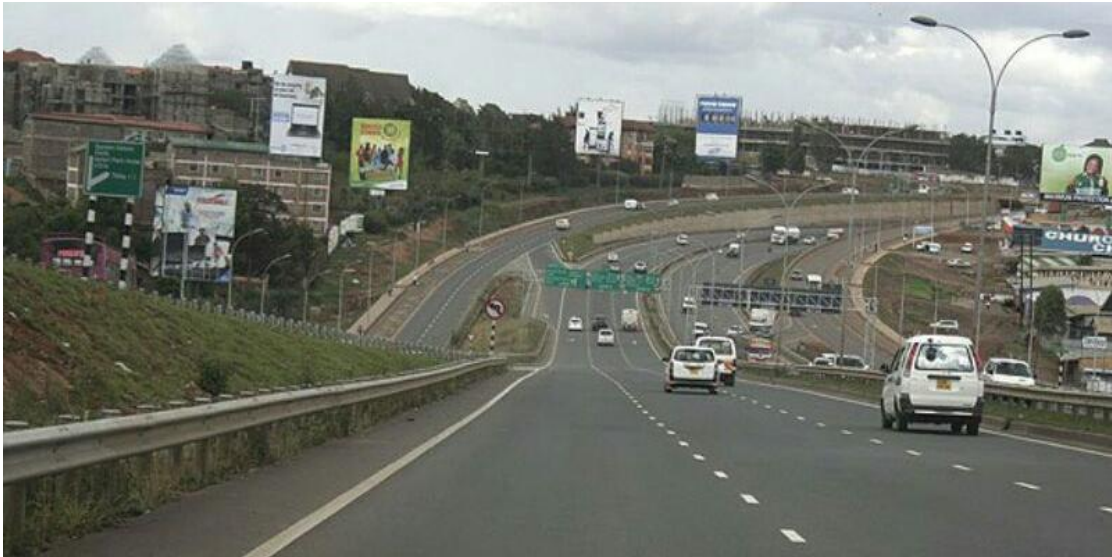
Plate 5.2 Six Lane Highway Between Allsops and Garden City Intersection Field Survey (2017)
