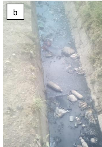
Plates 5.2 a,b,c: Illegal dumping and other poor practices of SWM often lead to unsightliness and clogged drainage channels in area of study.
