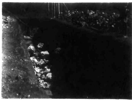
Excavation for Mill.
