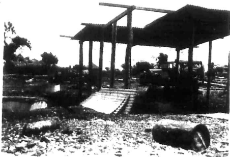
Construction work on Carlos Shaft.
