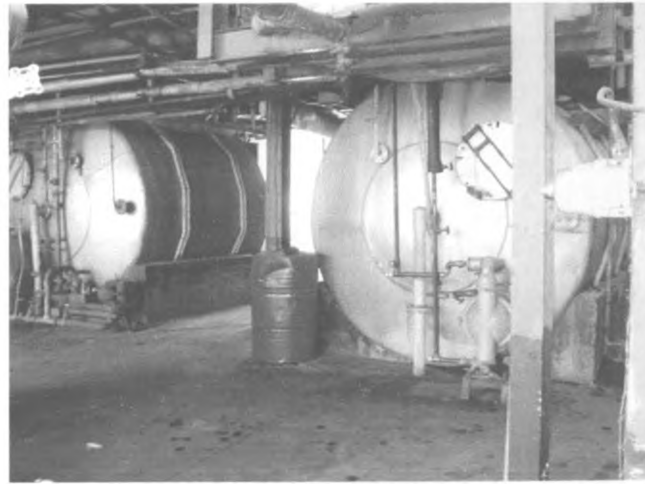
Figure 04. SST Storage and SST Miscellaneous Holding Tanks
