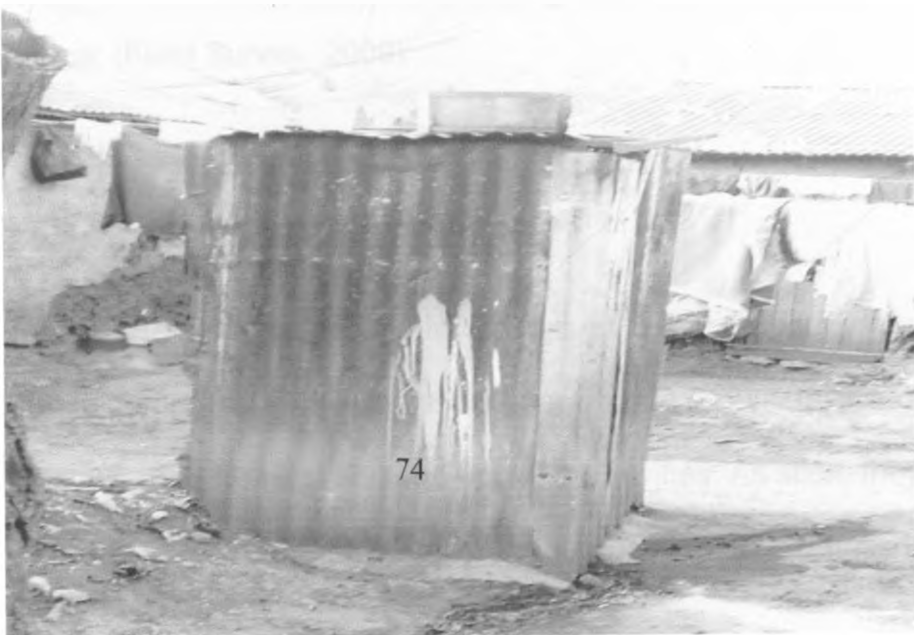
Plate 3: Iron sheet Super-structure Latrine
