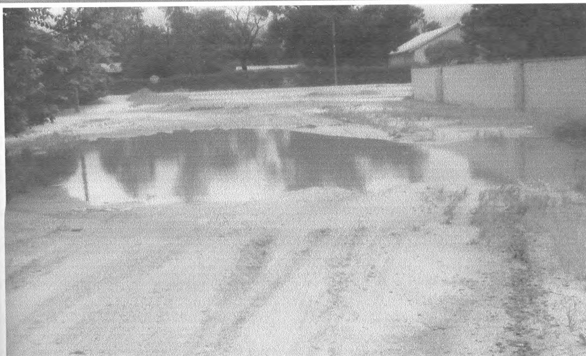
Plate 5: Poor road maintenance (Source: Field Survey 2010)
