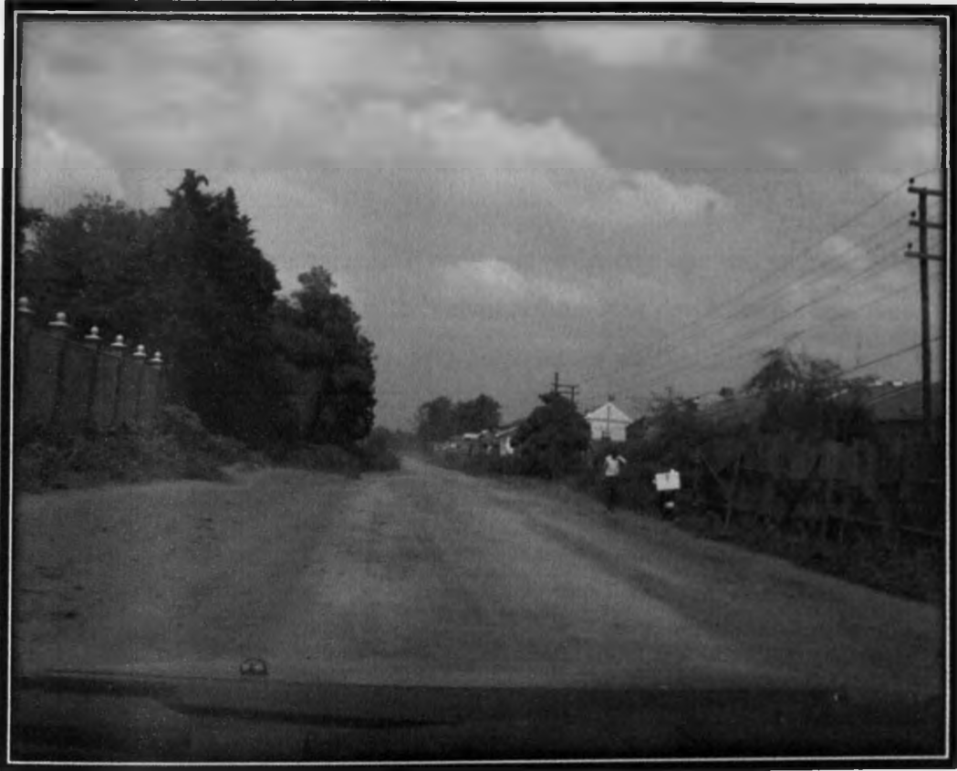
Plate 4-12: A section of the by-pass within Kileleshwa
