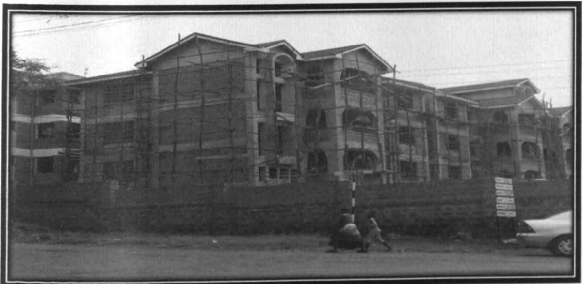
Plate 4-5: Apartments under construction within Kileleshwa
