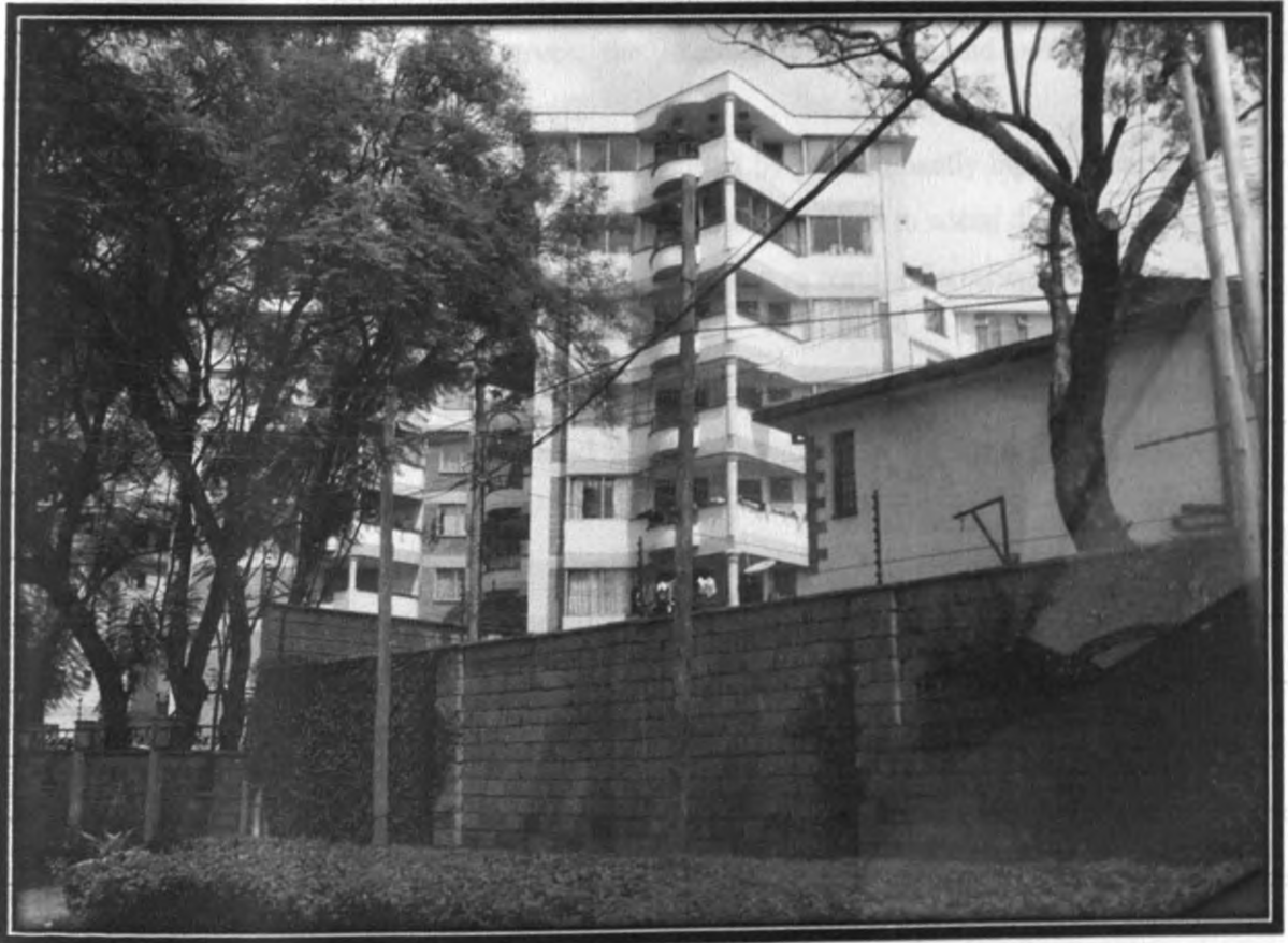
Plate 4-6: A building that exceeded the required floor limit
