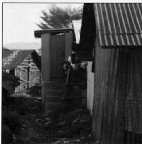
Figure 1.8 A Skyloo toilet in the Obunga settlement (Source: Adede, StAD student, 2007)
