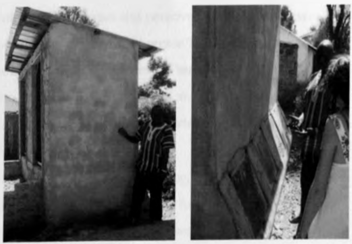
Figure 5.20 Incomplete communal EcoSan toilets put up at the Obunga Orphanage, located in Obunga Kasarani (Source: Researcher, March 2007)
