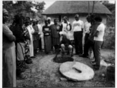
Figure 2.3 Construction of an Arborloo toilet (Source: P. Morgan, WSP-AF, 2005)
