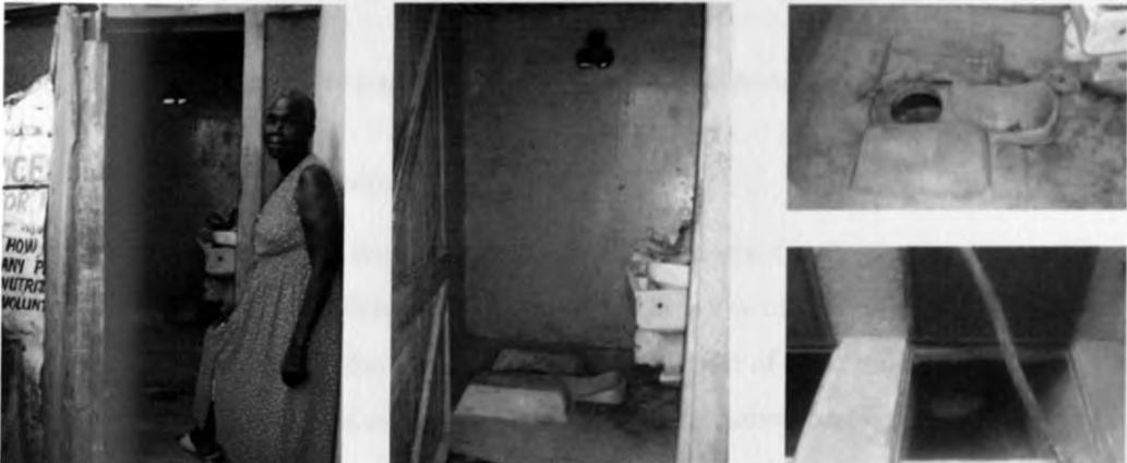
Figure 5.13 A household Ecosan facility showing the squat pan and emptying chamber situated at the rear of the facility (Source: Researcher, 2009)
