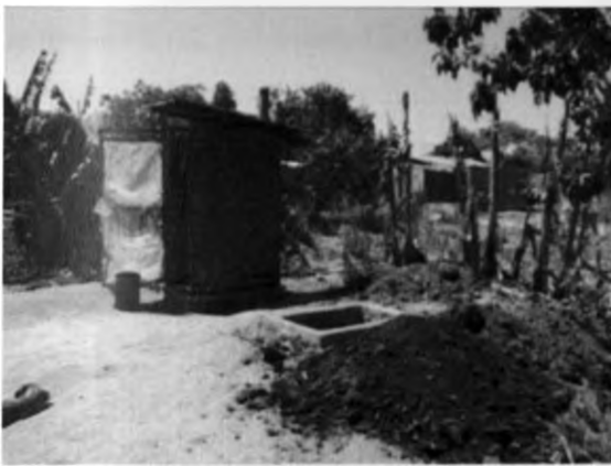
Figure 2.6 An example of Fossa alterna in Zimbabwe (Source: P. Morgan, WSP-AF, 2005)
