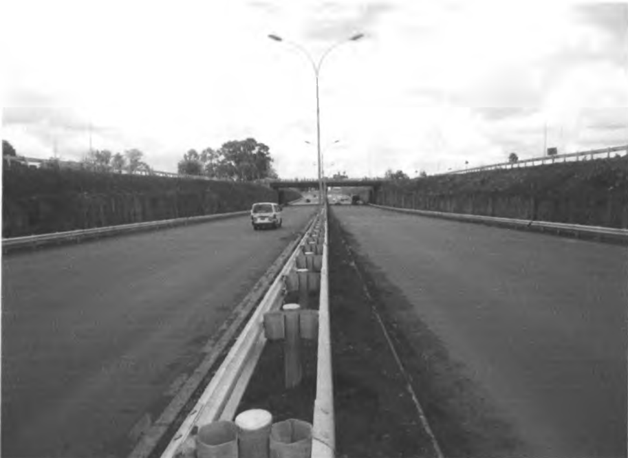
Plate 12: Deep cut section of the Nairobi-Thika Road (Km 6+550-km 7+730)
