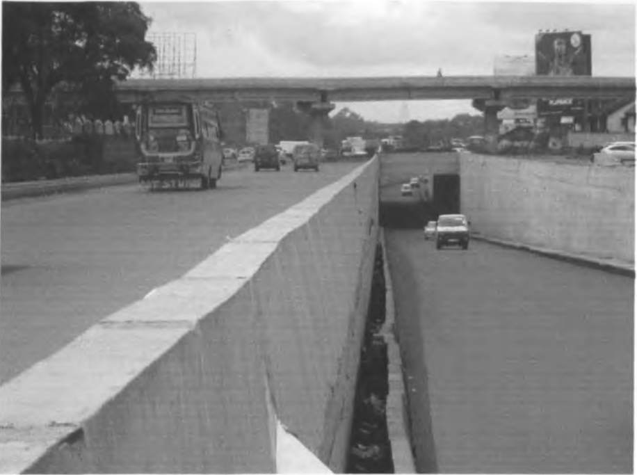
Plate 9: Pangani Underpass after construction (junction comprises of three levels)
