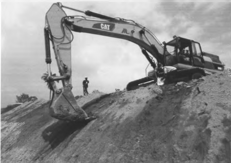
Plate 4: Scooping of soil sample @ km 3+100 using a track excavator
