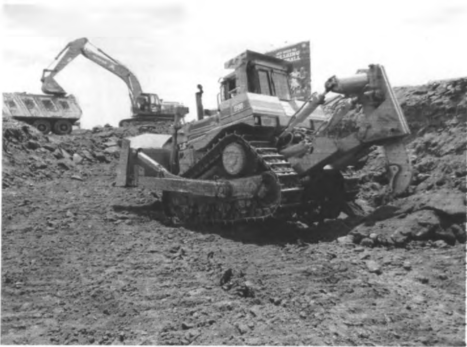
Plate 2: Excavation of material at Pangani Interchange
