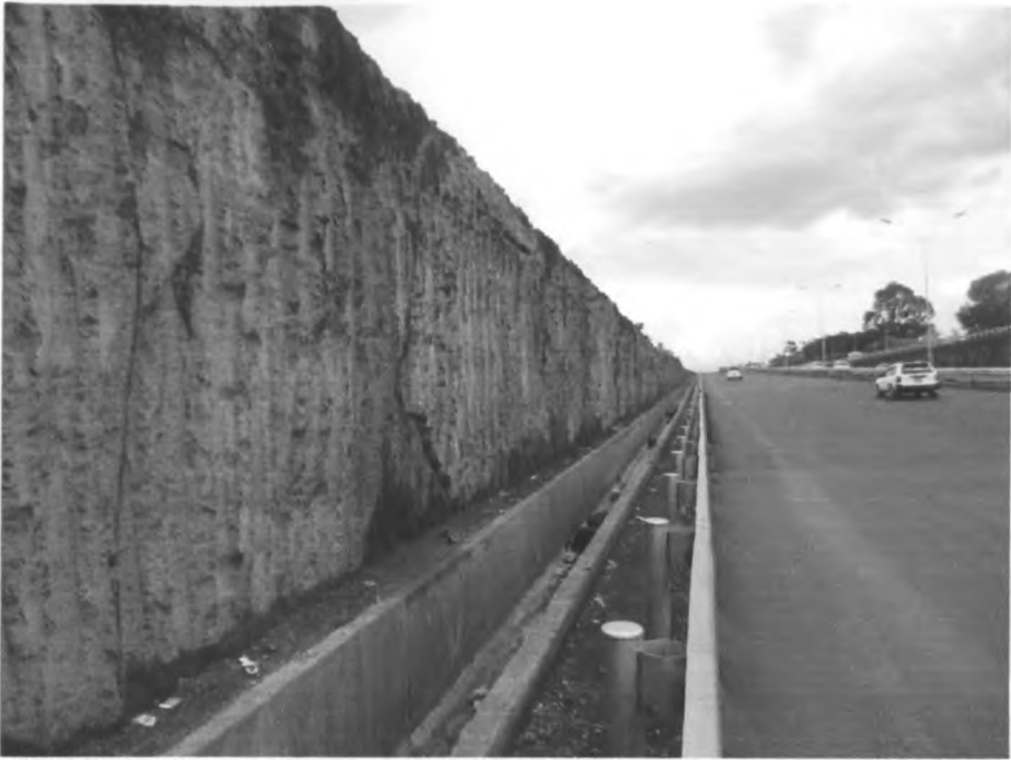
Plate 11: Showing embankment @ km7+100
