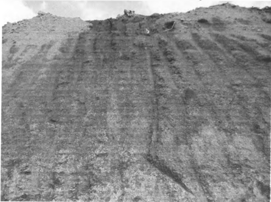
Plate 3: Section of embankment @ km 3+100 before sampling
