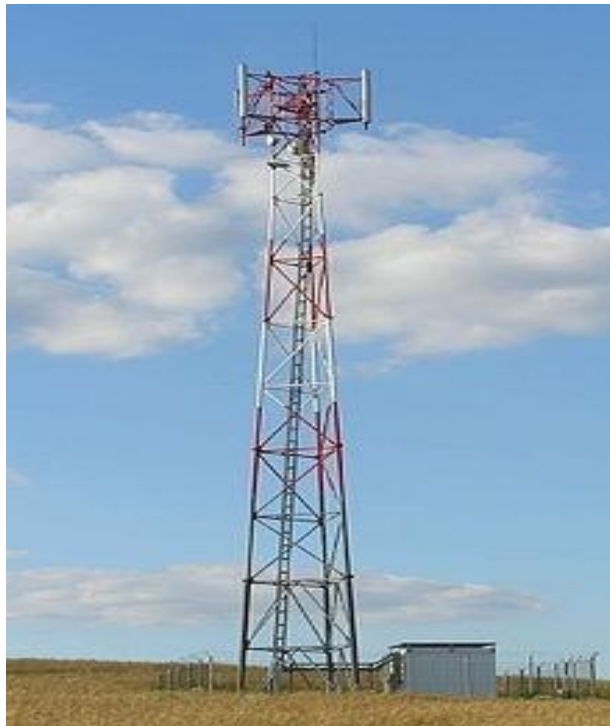
Figure 2.2 Typical Indoor BTS
