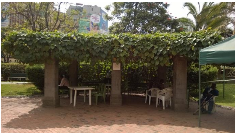
Figure 86: Pergolla made out of masonry pillars and covered in timber members
