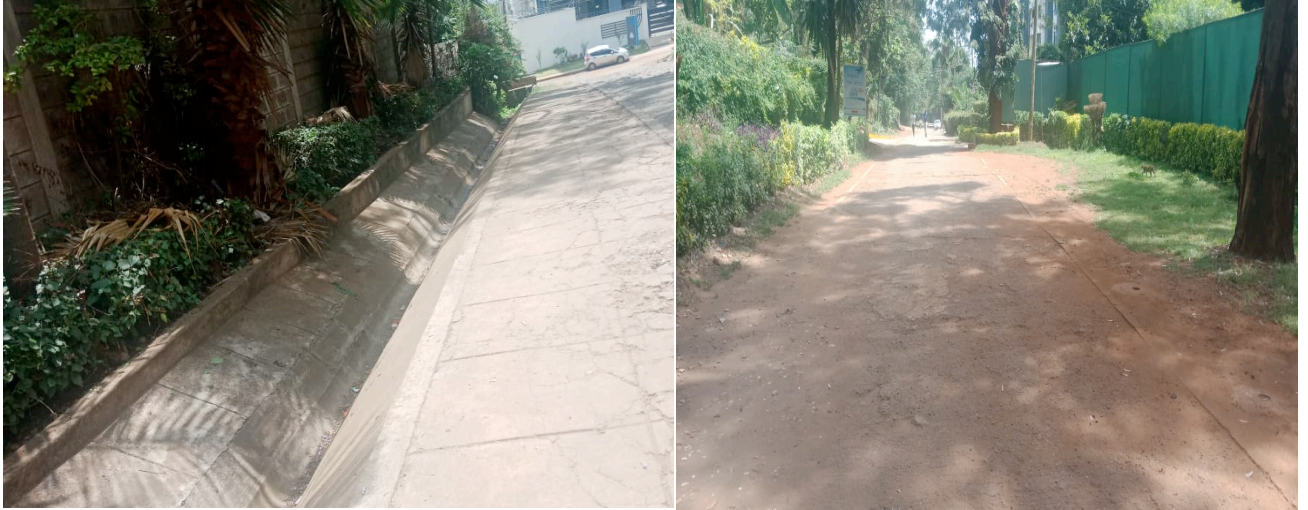
Plate 5.1: Section of Roads with Storms Drains
