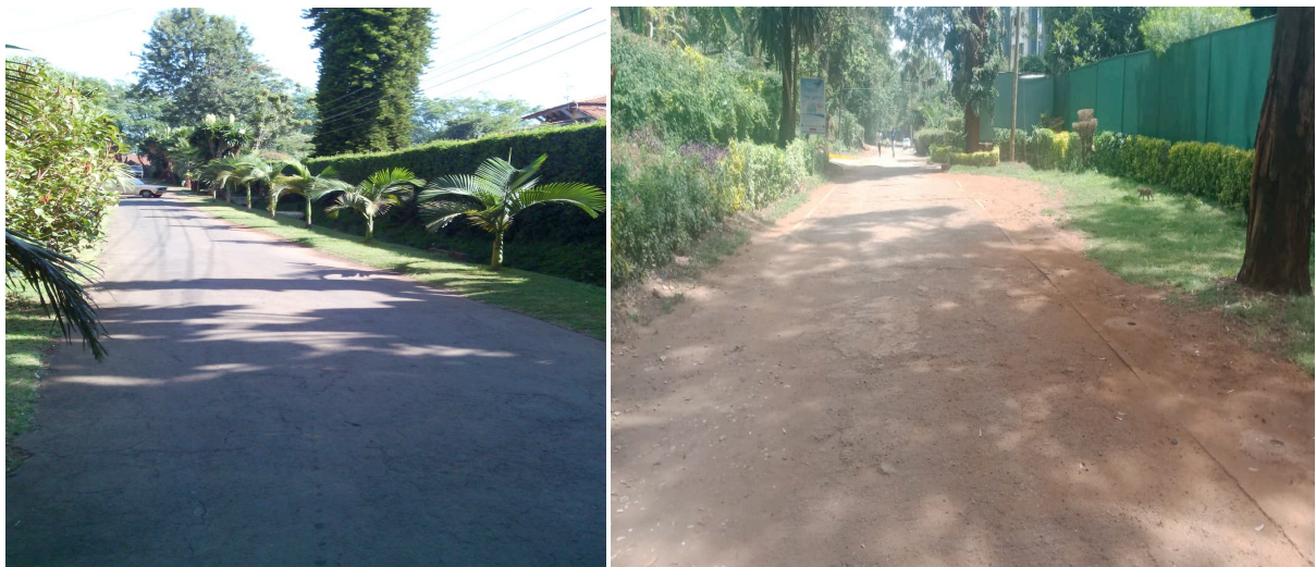
Plate 5.2: Access Road in Riverside Neighbourhood
