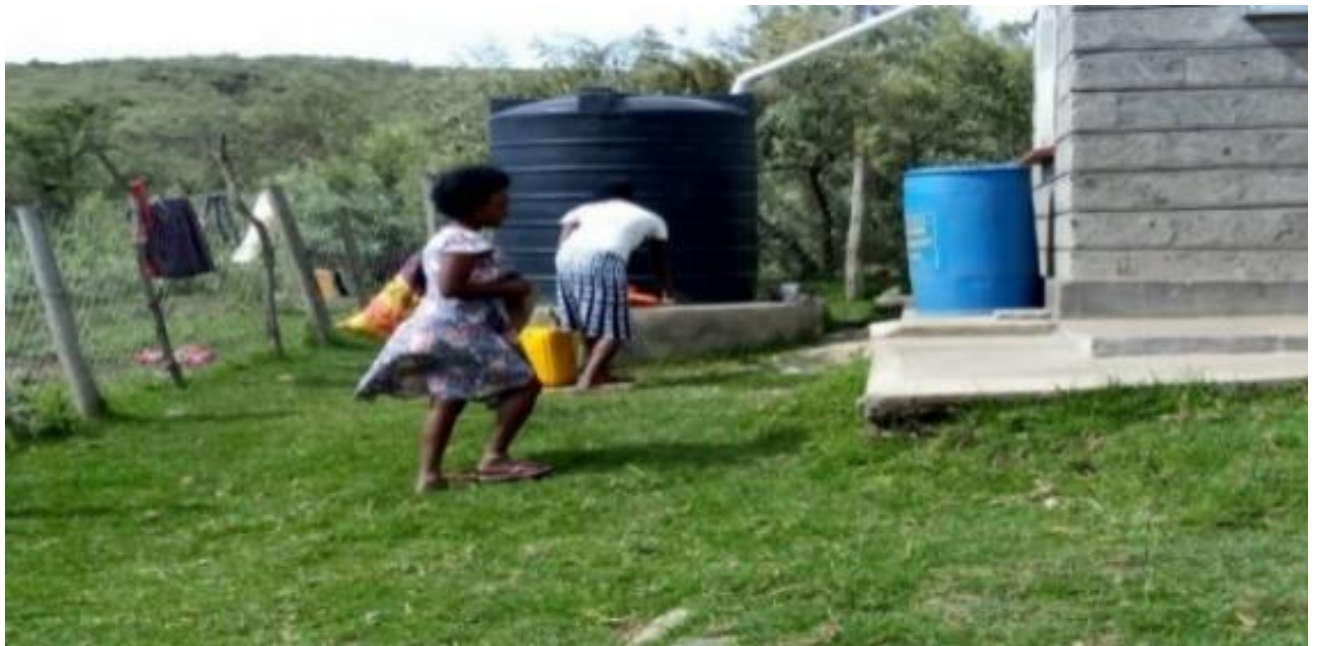
Figure 4.4: Water Tank for rainwater collection. Source: From Researcher's photos gallery.
