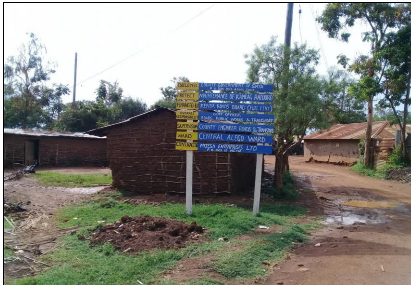
Figure 20 Proposed Maintenance works of Kamlag – Ratuoro Bitumen Road
