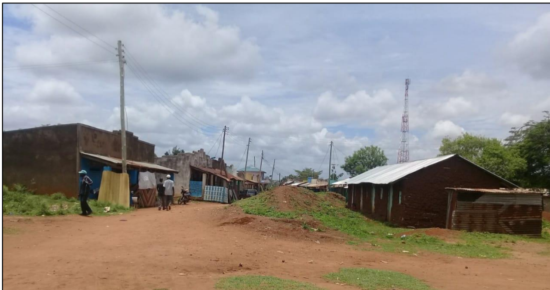
Figure 30: Permanent and Semi-Permanent Structures at Boro Market
