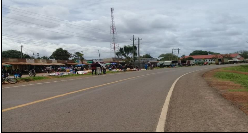
Figure 18: C29 Bitumen Road from Siaya Town to Port Victoria at Boro Market
