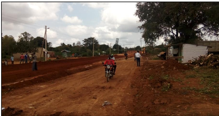
Figure 19: Ndere – Boro Bitumen Standard Road Upgrade
