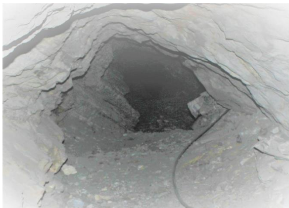
Ready for blasting
