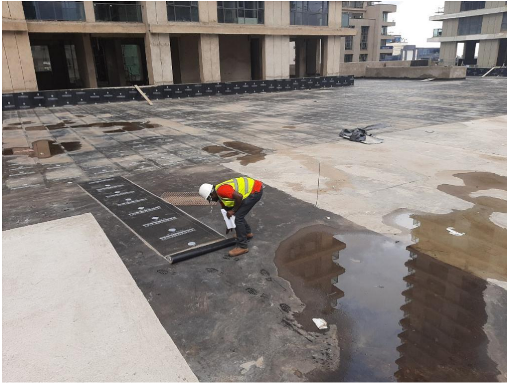
Photo 6; on-going green roof installation of the GTC vegetated roof
