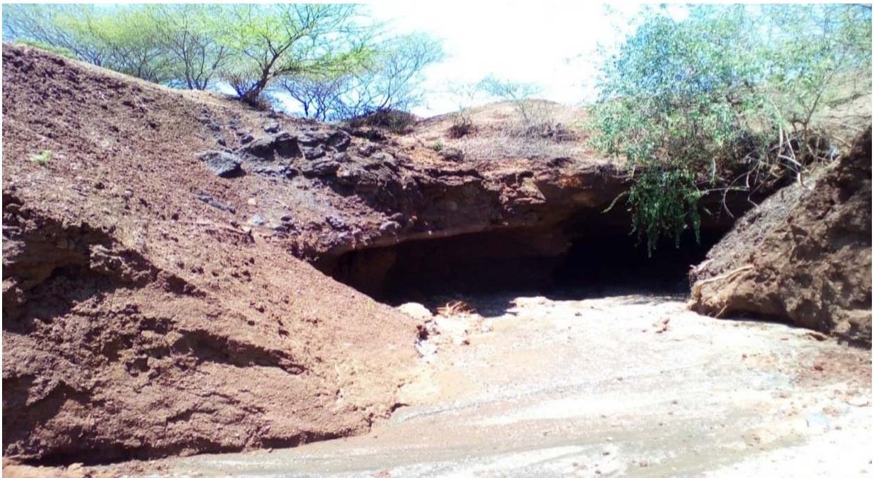
Figure A 4: Erosion gully developed by seasonal river flash floods
