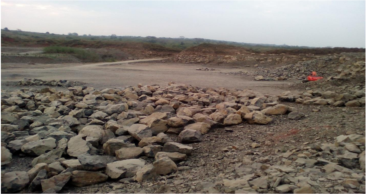
Figure A 5: Quarry excavation site at Ebul bul
