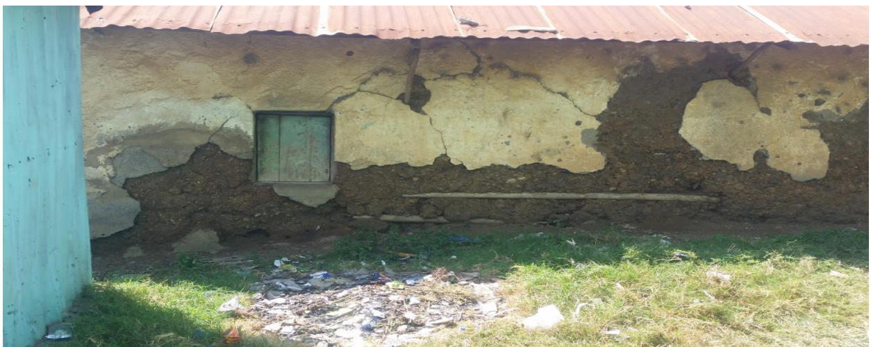
Figure 4.1 Household wastes behind the building
