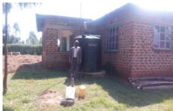
5.2 Rainwater harvesting in Kamusinga Location
