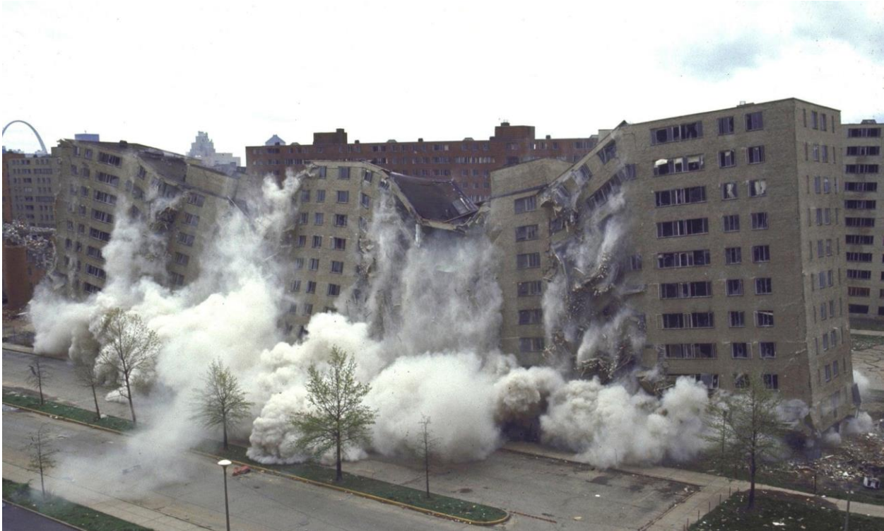
Figure 7: Demolition of Pruitt Igoe 1972
