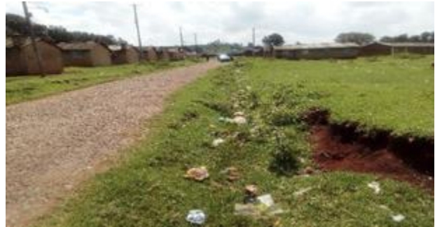
Figure 14: Access routes in disrepair
