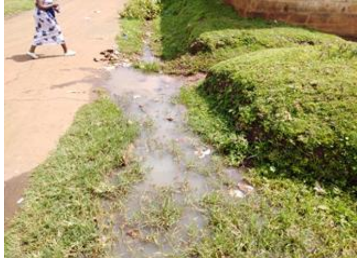
Figure 17: Poor run-off management
