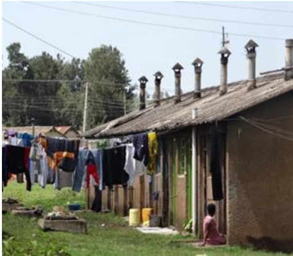
Figure 29: Row Housing with Asbestos roofing
