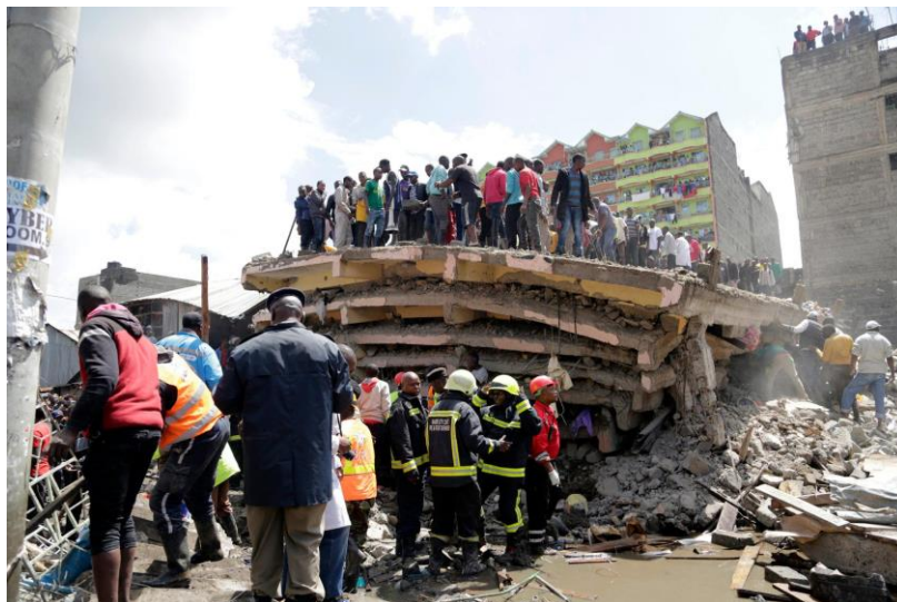
Figure 3: Collapsed building, Kayole Nairobi.
