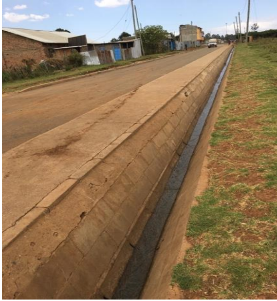
Figure 4.11: Open paved stormwater drains, tarmacked road and electricity in Munyaka settlement.
