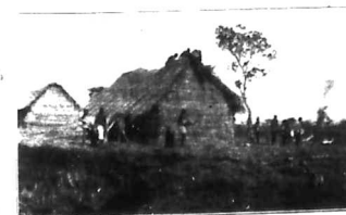
Bathouse at Marwa, being constructed by Messrs. H. F. Ward & Co.
