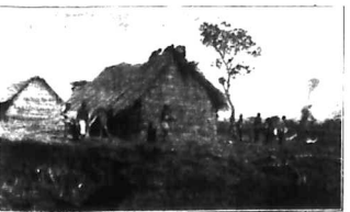
Bathrooms at Mas'wa, being constructed by Messrs H.F. Ward & Co.
