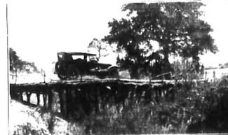
New Utungole Bridge
