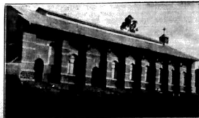
Built by Natives: New Church of the Catholic Mission at Mombasa completed in 27 months. Local burnt bricks (200,000) and local acacia timber were used. The church seats 1,200.
