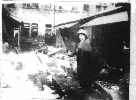
The view from the bank of the premises, before the fire had taken a strong hold of the lower floor. A narrow escape from death. One is depicted shortly after striking a vessel in a narrow building.
