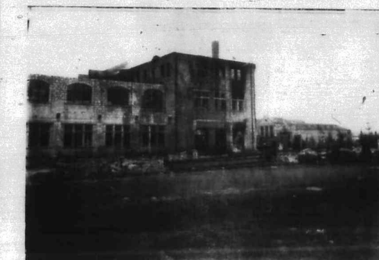
The entrance to the building after the fire had been put out.
