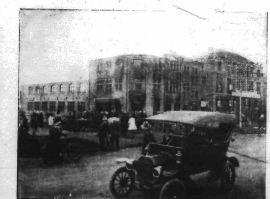
The crowd inspecting the damage and enquiring as to the results of the search for the body of the victim (Mr. Cowan). The body was ultimately discovered under boring done in a corner of this ship having the main entrance
