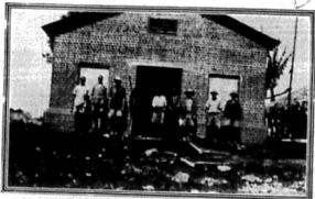
A new Kikuyu House nearing completion.
