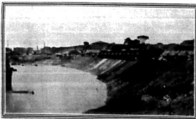
(1) The quay wall of the fourth deep water berth at Kilindini. (2) The work of filling in for the fifth berth. Pictures: Hon. T. J. O'Brien.
