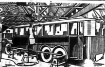
A 30-seater bus being finished in Duro white and red.
