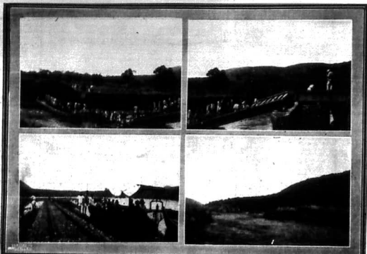
Four scenes of the disastrous floods on the Central Railway, Tanganyika, which have resulted in a loss of revenue amounting to £8,000 a week. The bottom left hand picture shows one of the launches used to transport passengers on the great inland lake formed by the abnormal rains. Photos: M. G. de Courcy-Ireland.
