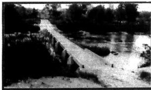
The Athi River Bridge, near Schabas. Photo: F. E. Holland, K.M.
