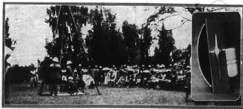
Laying the foundation stone of the New Central Office of Government at Nairobi. Photo: Bode, Nairobi. The boys used in connection with the first two ceremonies and the silver hammer in the frame of a towel all presented to His Excellency were made by James Laidlaw, Nairobi.
