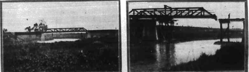
The railway bridge over the Nile River on the Nile-Kinshasa construction.
