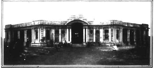
THE GOVERNMENT BUILDING, NAIROBI.
